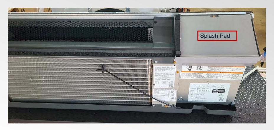
2. Using a ¼ inch nut driver or slotted head screwdriver remove the 3 screws from splash pad cover. Remove the splash pad from the Amana PTAC unit.
