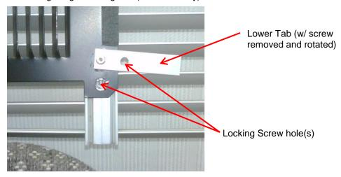
With the grill fully outside of the unit, raise/slide the grill so the top flange on the back of the sleeve slides between the top mounting brackets and the vertical struts. Push up to fully seat the flange.
